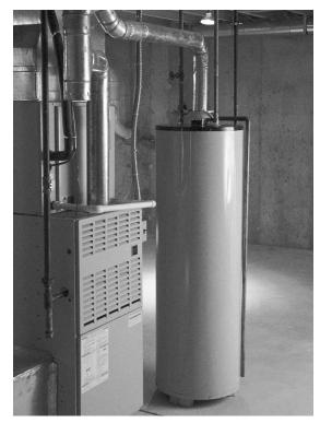
Atmospherically vented appliances, such as this water heater, should be direct-vented to minimize carbon monoxide exposure.
