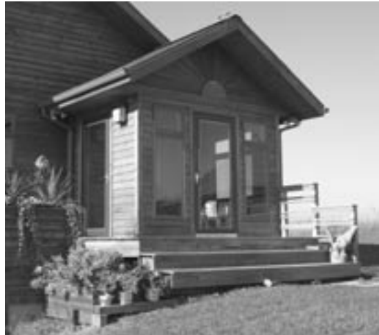
(top) A passive solar-heated vestibule in the Rezabek/Strous house functions as an “airlock” that reduces cold air infiltration. The long window on the left faces south and heats the stone tiles inside.
