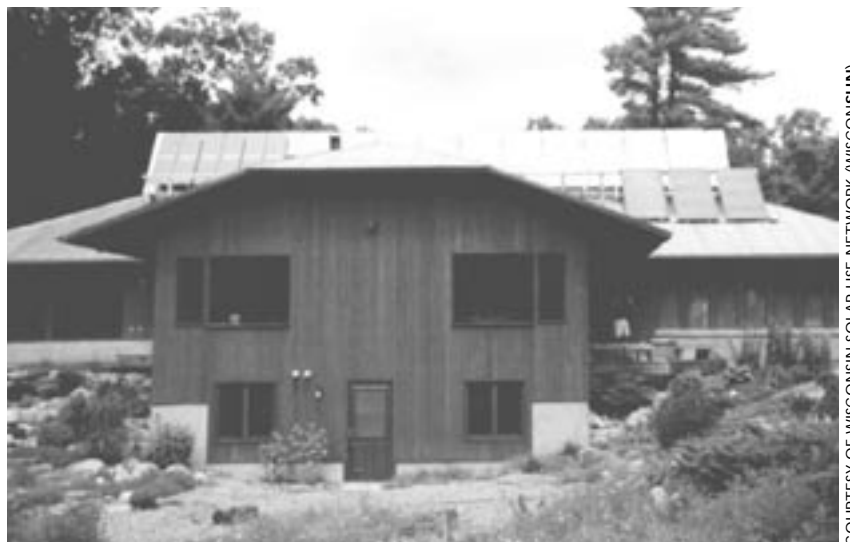
(below) The Davenport home combines passive and active solar heating technologies. South facing windows heat the house during the day while ten roof-mounted solar collectors heat a fluid that flows beneath the house and warms 200 tons of sand and concrete. By nighttime, the thermal mass is warm enough to heat the house by radiating up through the floor.
