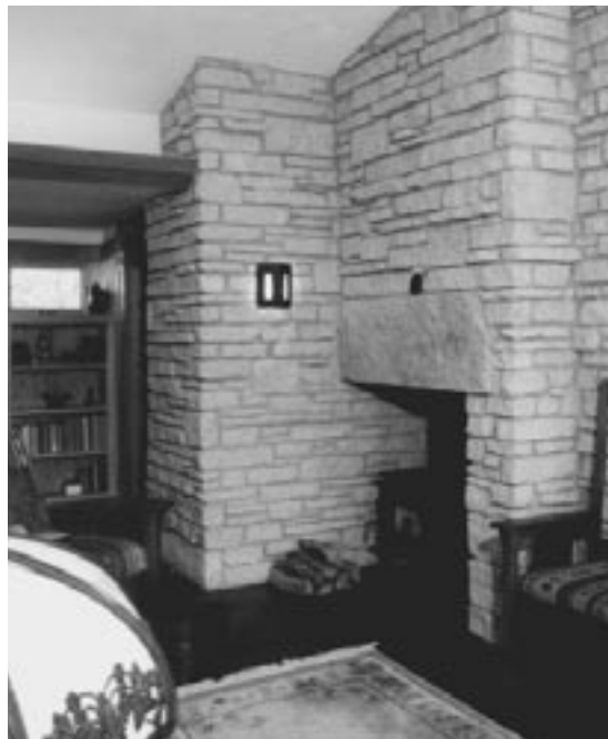
(left) The masonry fireplace in the Hoerr home is fitted with a high efficiency wood burning stove. As exhaust rises through the masonry, the stones warm and radiate heat to the living room, supplementing the heat provided directly by the stove.
