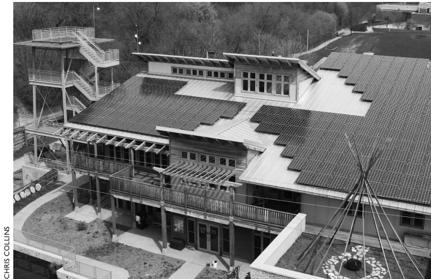
(top) The Urban Ecology Center in Milwaukee, Wisconsin features a fixed-mounted 44.4 kW system on its roof.
