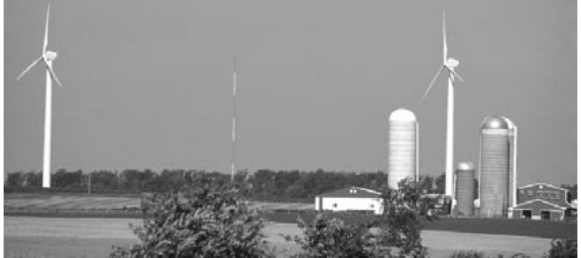
Wisconsin Public Service has installed two Tacke 600 kW Turbines on the Zirbel Farm in Brown County, Wisconsin.
