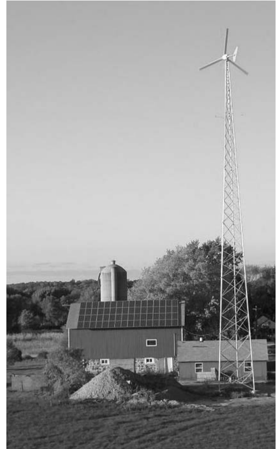
A combined solar electric and wind turbine system at TDL Electronics near Racine, Wisconsin. The 10-kW wind turbine and the solar electric system powers several homes in the neighborhood.
