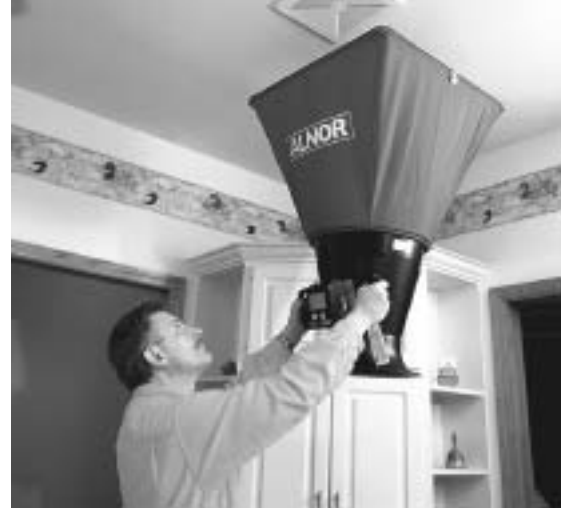
An HVAC contractor conducts an exhaust ventilation test to ensure the system performs effectively.
